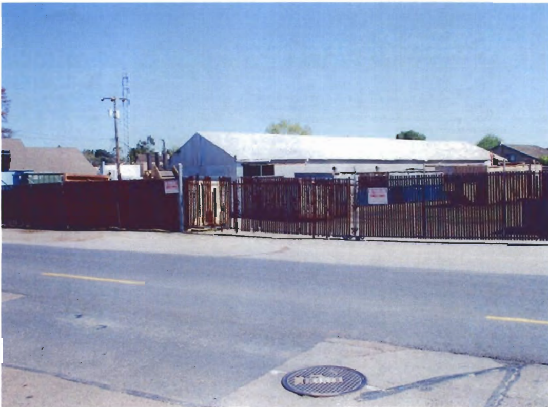
Photograph 2 – View to the southwest of the shop building
