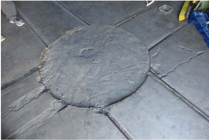
9. View of track feature inside building
