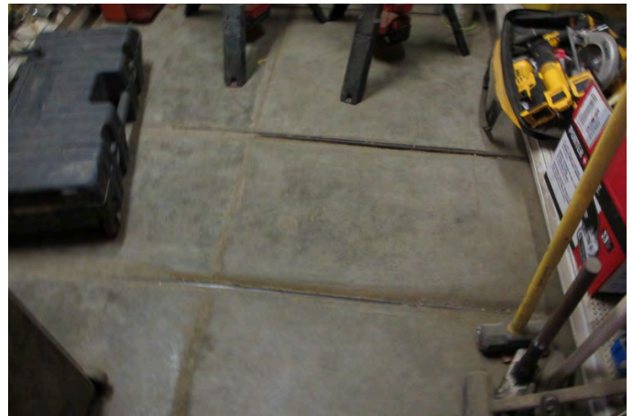
12. View of track feature inside building
