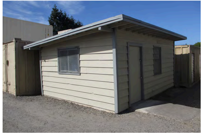
14. View of small storage structure
