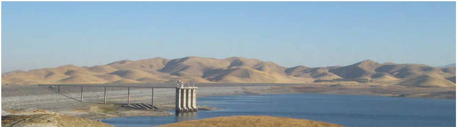
San Luis Reservoir, October 2015
