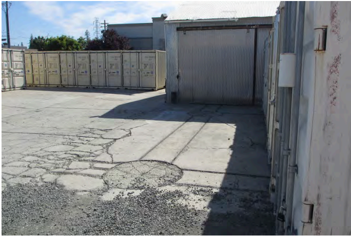
13. View of track feature on outside of building
