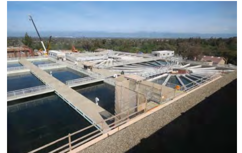
Rinconada Treatment Plant photo: SCVWD
