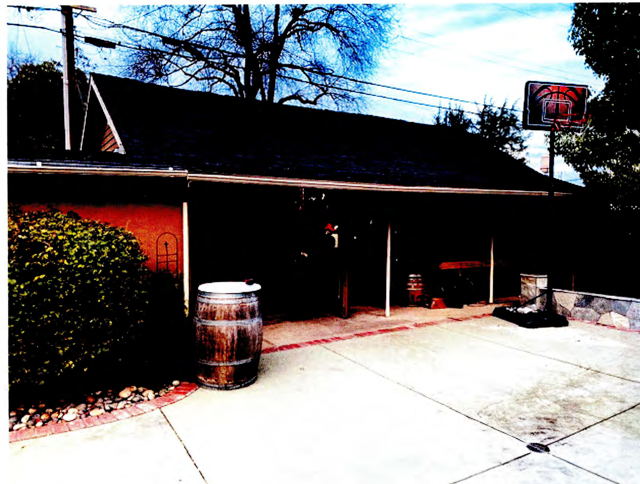
FRONT MIDDLE OF GARAGE
