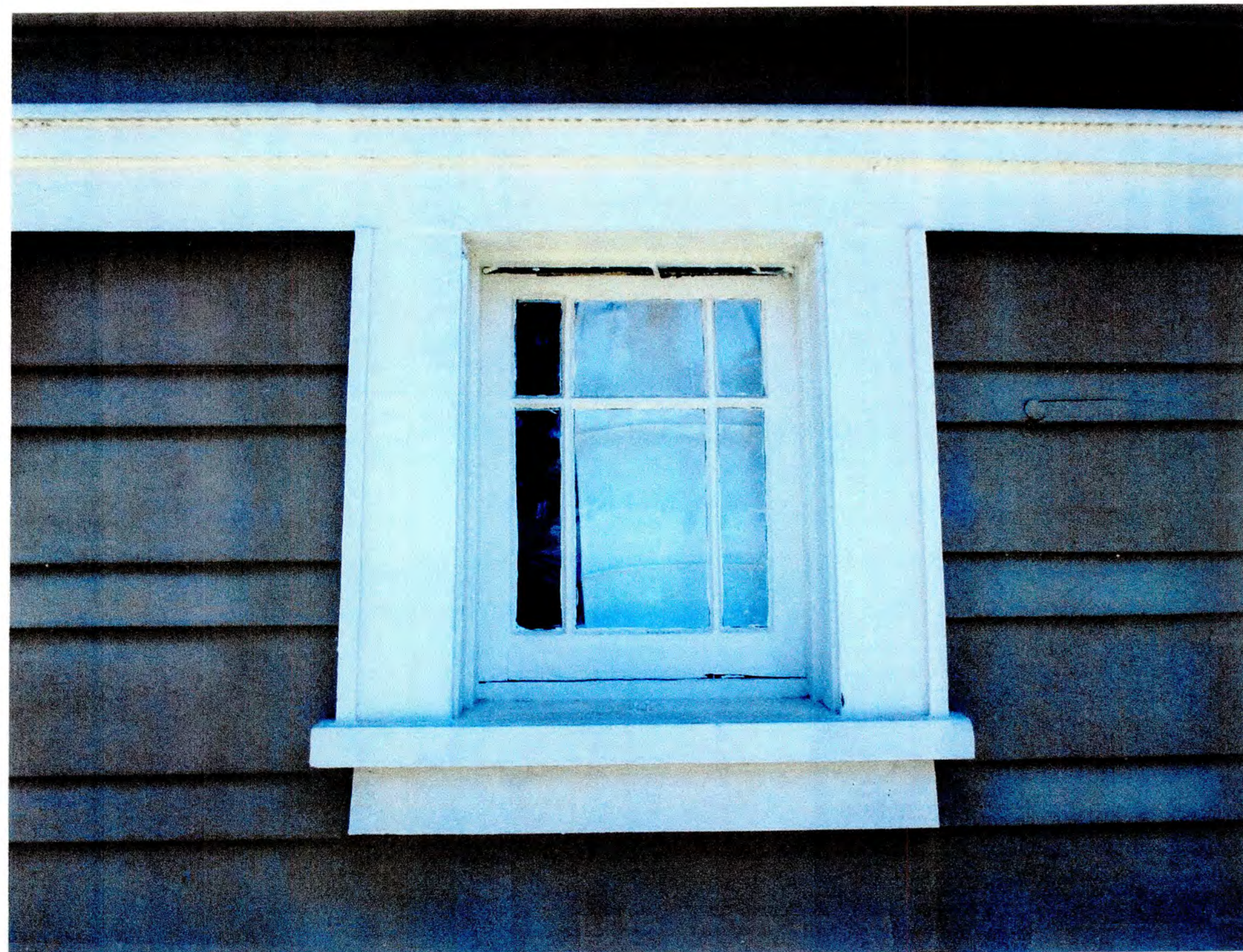
ORIGINAL WINDOW DESIGN (1 OF 4 ORIGINAL REMAINING)
