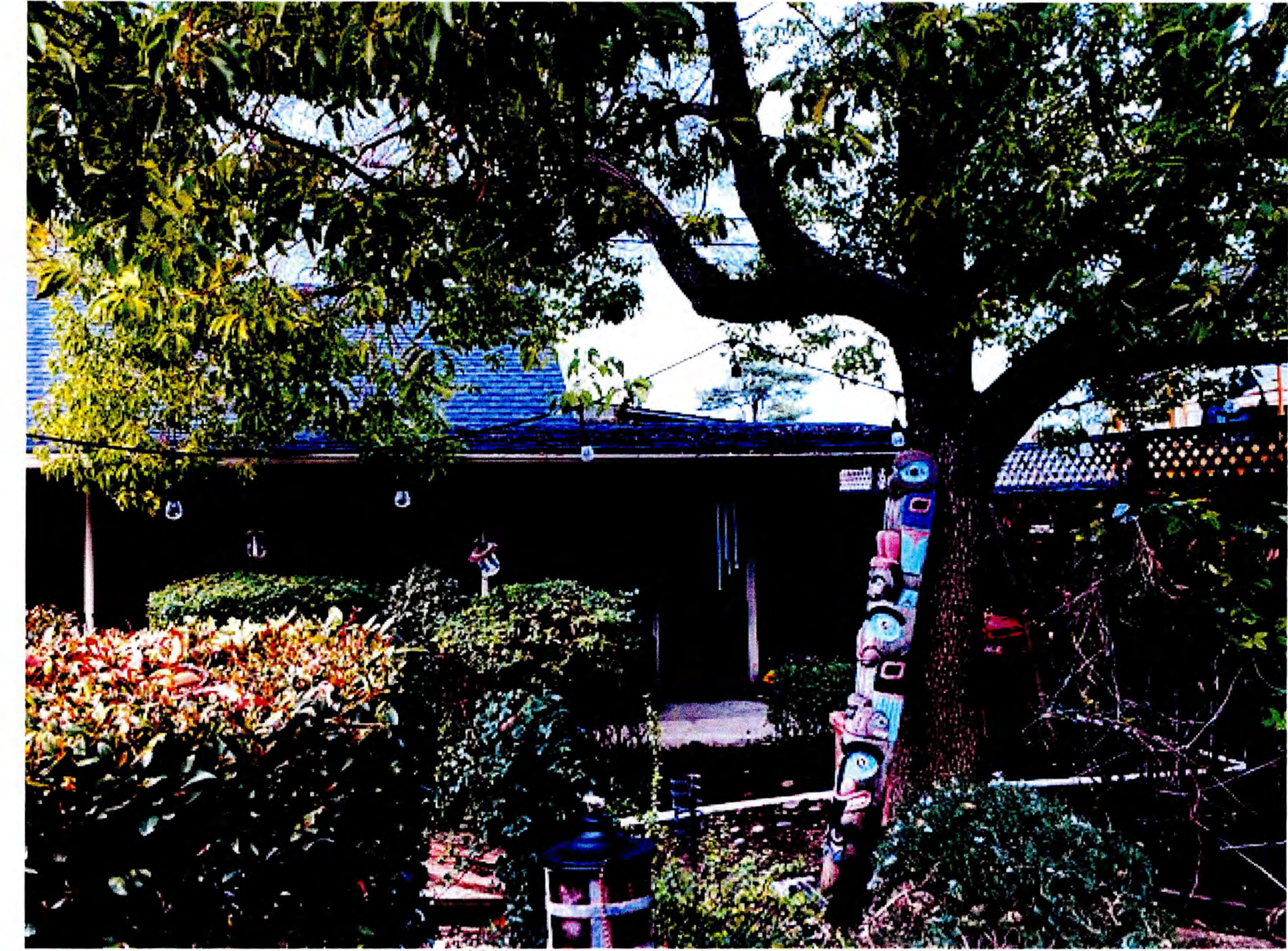
FRONT RIGHT SIDE OF GARAGE
