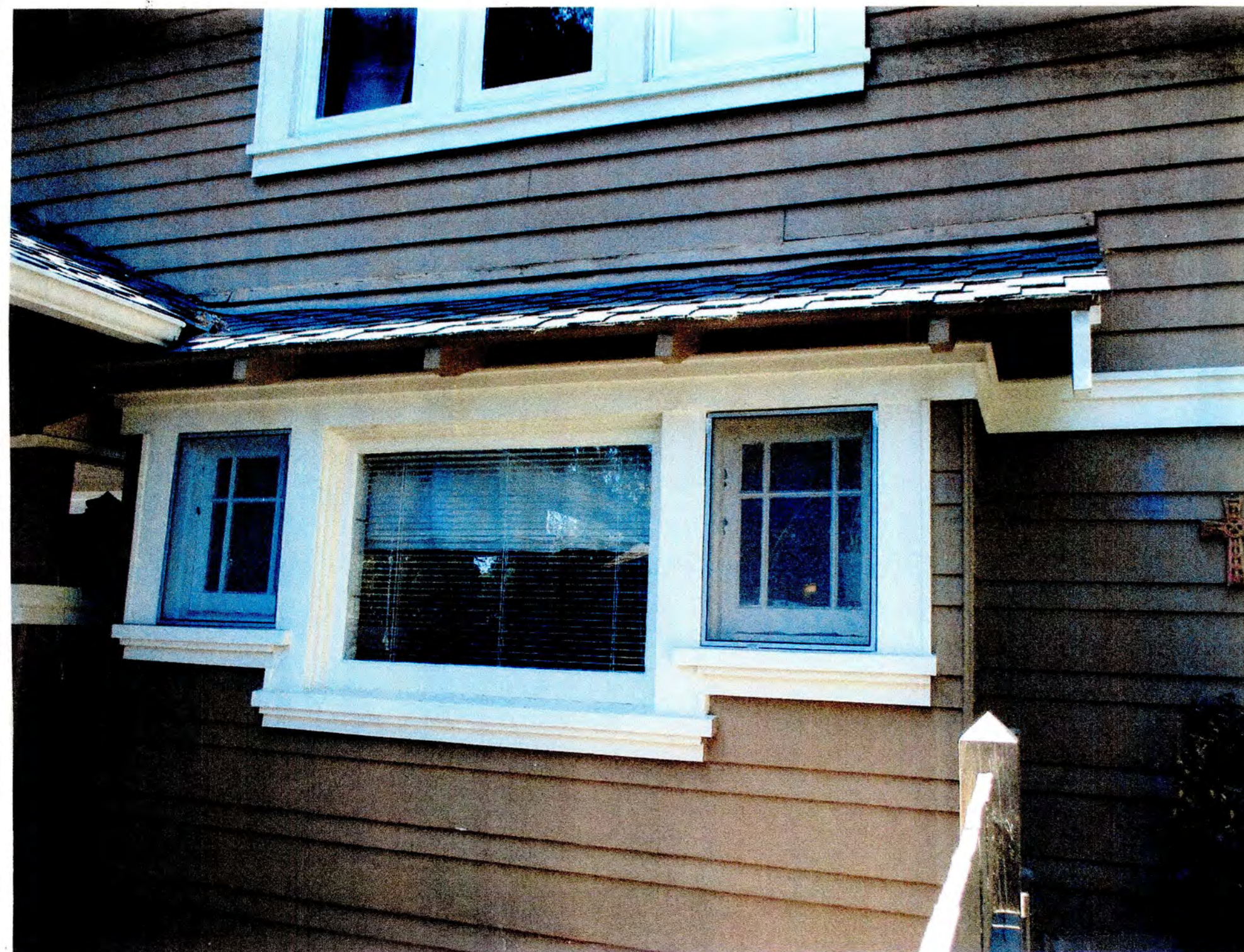
ORIGINAL WINDOW DESIGN (3 OF 4 ORIGINAL REMAINING)
