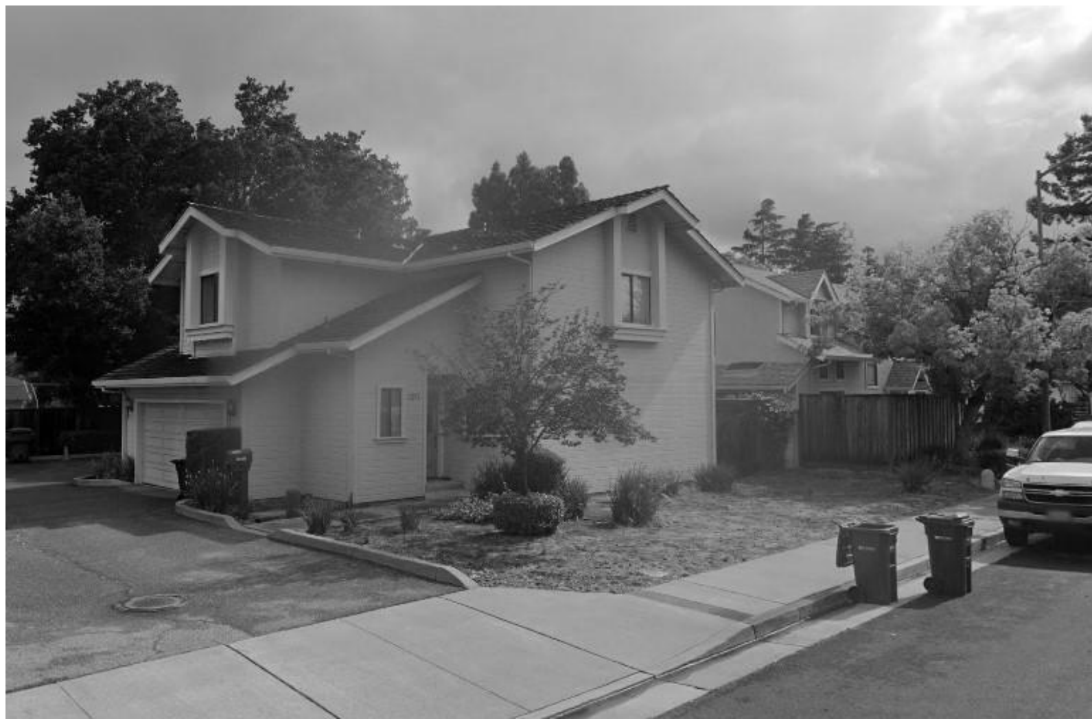
1204 SMITH AVE, 2 STORY WALLS, MIX OF GABLE AND SHED ROOFS
