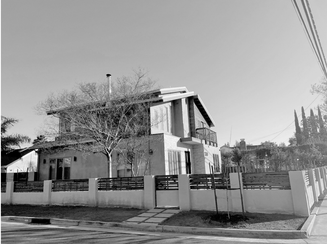
1360 BURROWS RD. MIXED ROOF PITCHES, MIX OF GABLE AND SHED ROOFS, APPLIED MATERIAL FINISHES, 2-STORY WALLS
