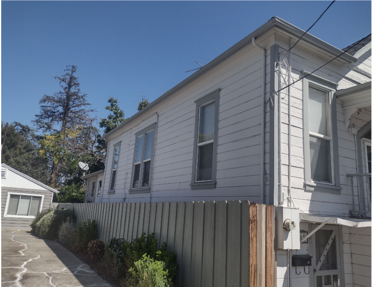
Figure 6. West Facade, facing northeast
