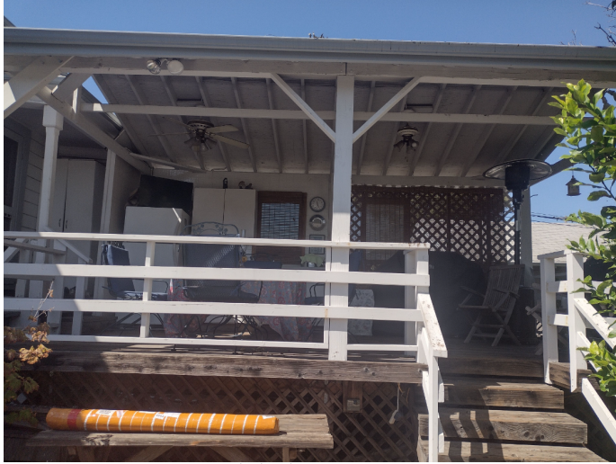
Figure 8. Rear covered deck, view west
