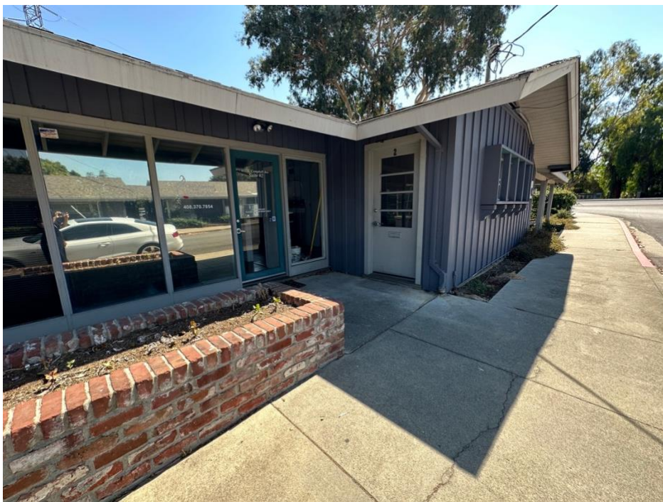
653 Unit 2 Exterior Facing Poplar Ave (Image 4)
