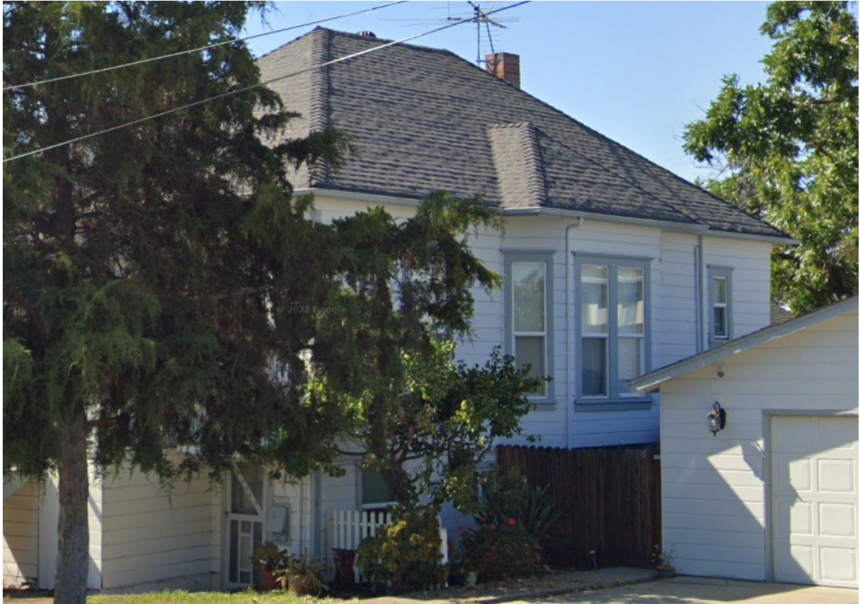
Figure 9. East facade, view northwest
