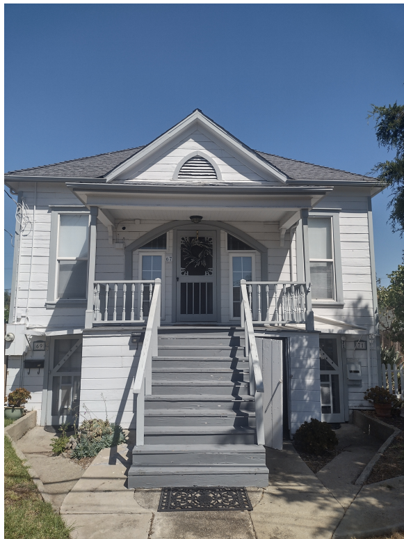
Figure 3. South facade, facing north
