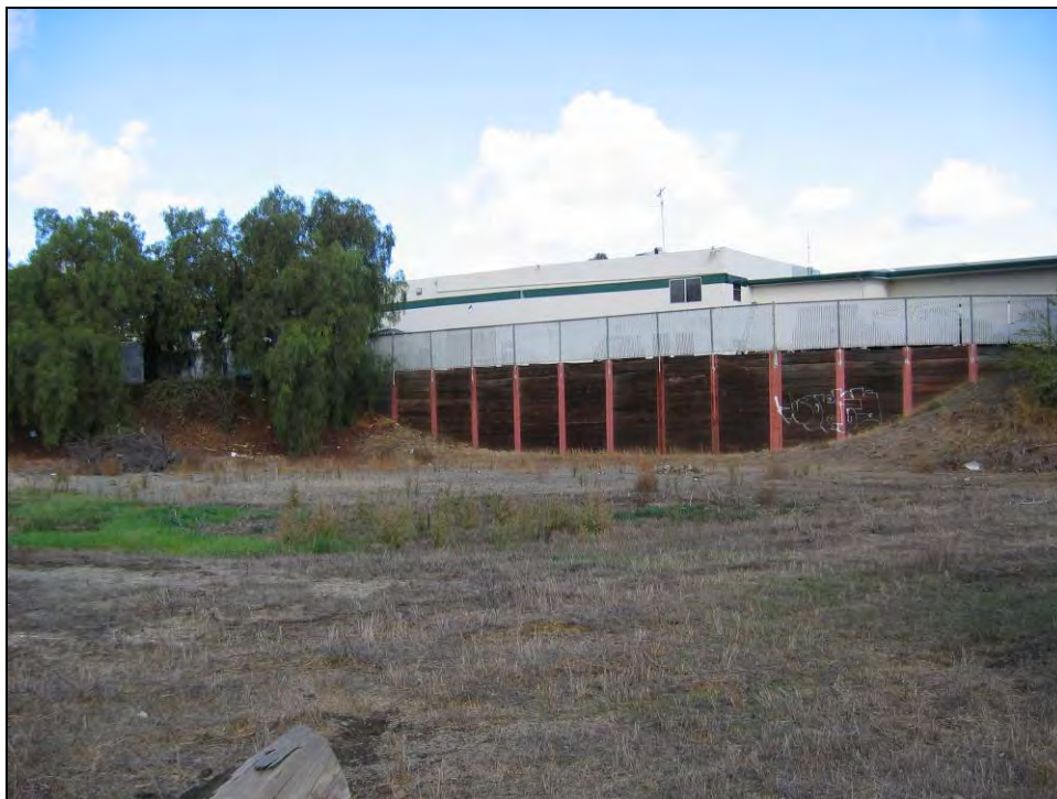
VIEW OF THE SITE LOOKING NORTHERLY
