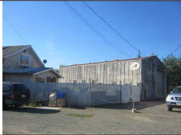
View of entrance to 328 and 330 Railway Avenue from the north
