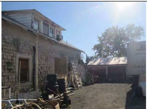
View of the south side of 328 Railway Avenue
