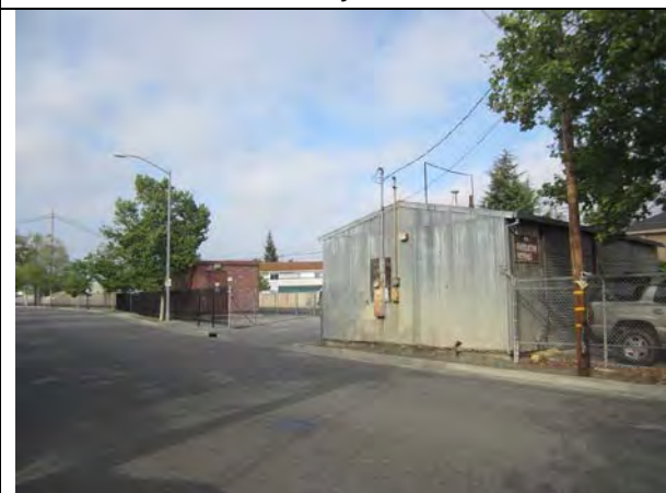
View of 261 Railway Avenue northeast
