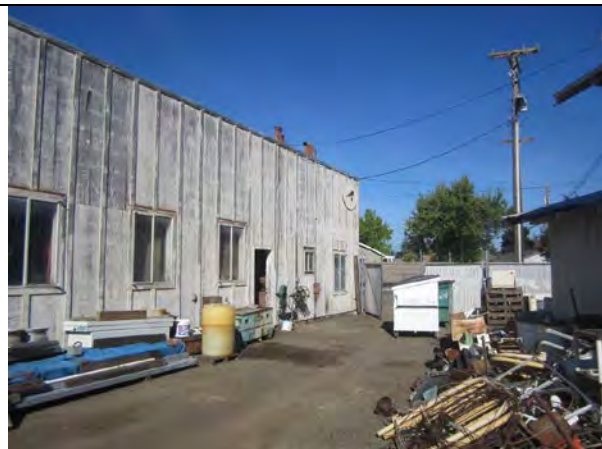
View of the north side of 330 Railway Avenue
