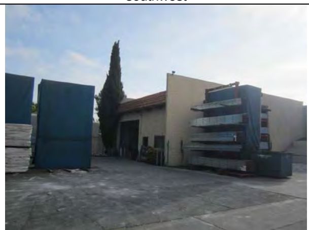
View of 232/238 Railway Avenue from the southwest
