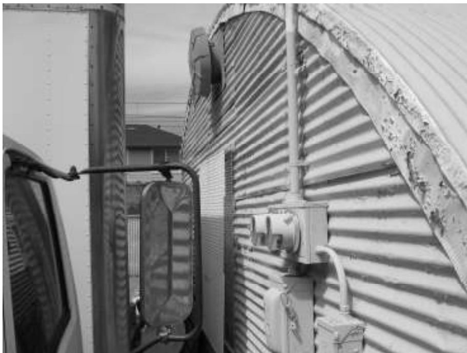
Photo 5: Oblique view along the north façade.
