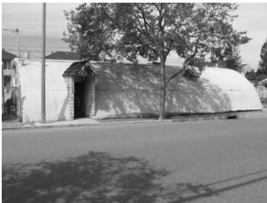
Photo 1: View of 241 Railway Avenue from the northeast.
