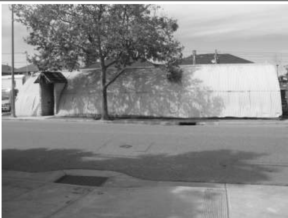
Photo 2: View of the structure from the southeast.
