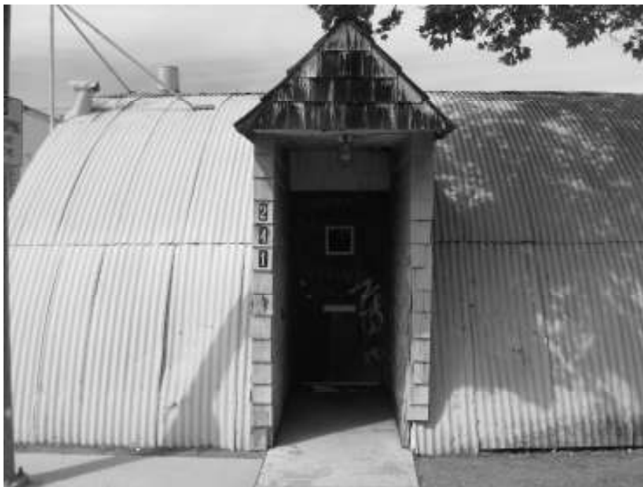
Photo 3: View of the gabled entry.
