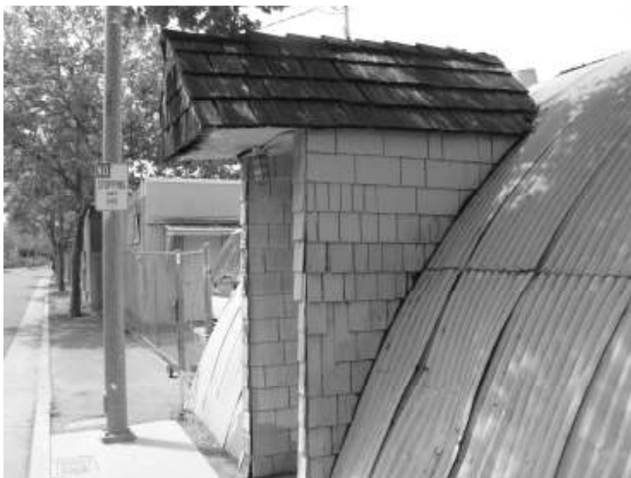
Photo 4: Side view of the gabled entry.
