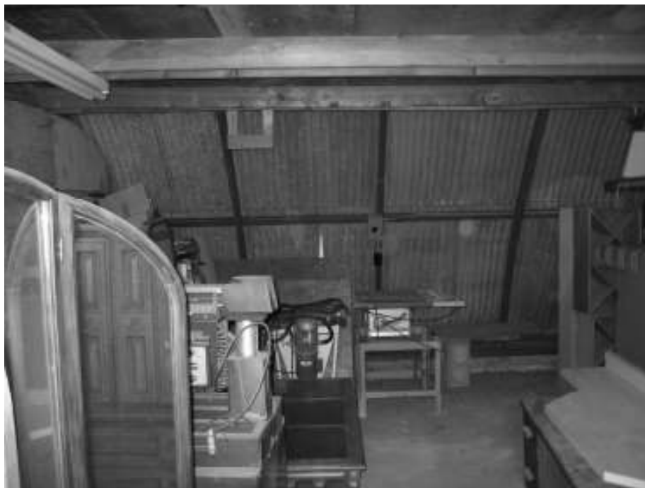
Photo 9: Interior view of the unfinished garage area.
