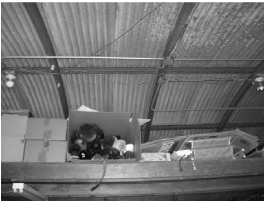
Photo 10: View of the barrel vault ceiling.
