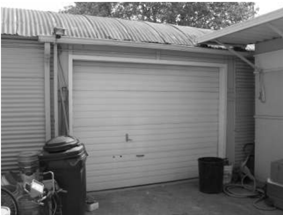
Photo 8: View of sliding door entry on rear façade.
