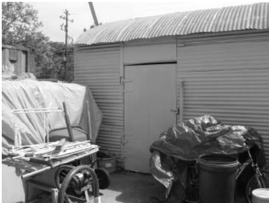
Photo 7: View of vertical wall along the rear façade.
