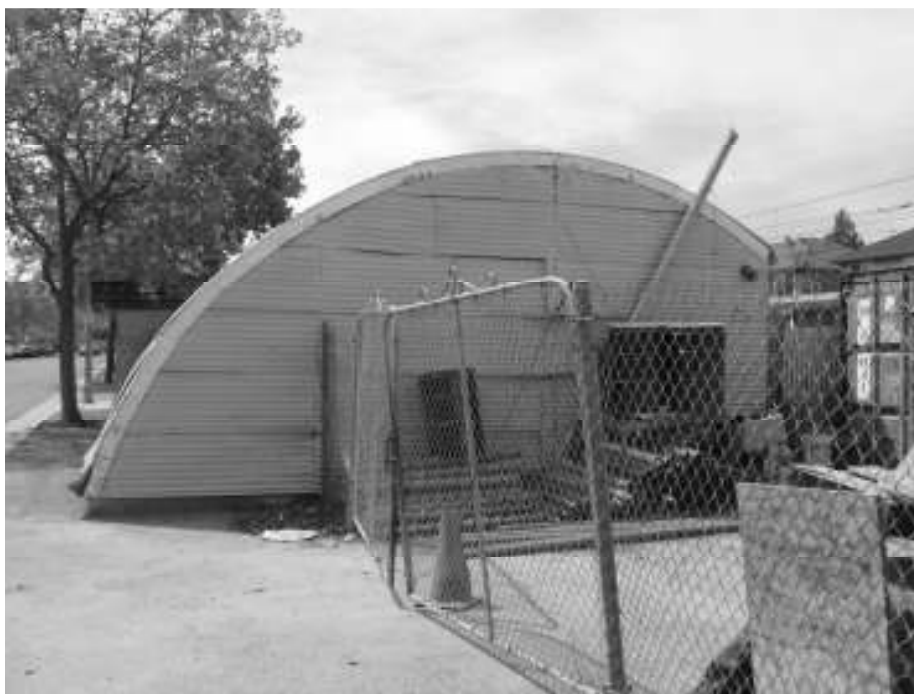
Photo 6: View of the south façade, note truncated arch.
